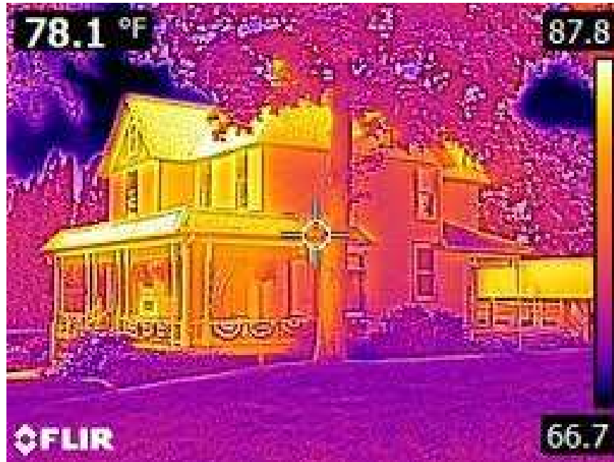
In this old house, the exterior cladding is HOT
