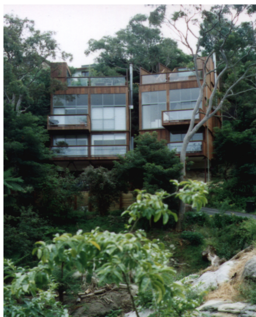
Housing can sit above the ground plane with pole construction or be grounded with localised areas of excavation
