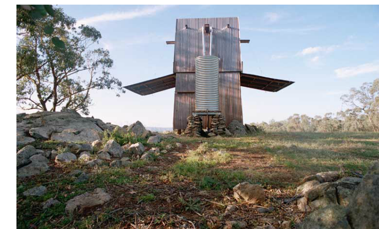
small above ground water tank integrated with the house design
