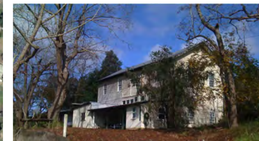
5 Old admin office (former grafting shed) to be reused as a cafe and local store
