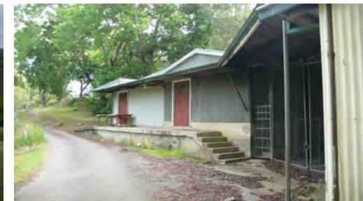
5 Siding associated with the old admin office
